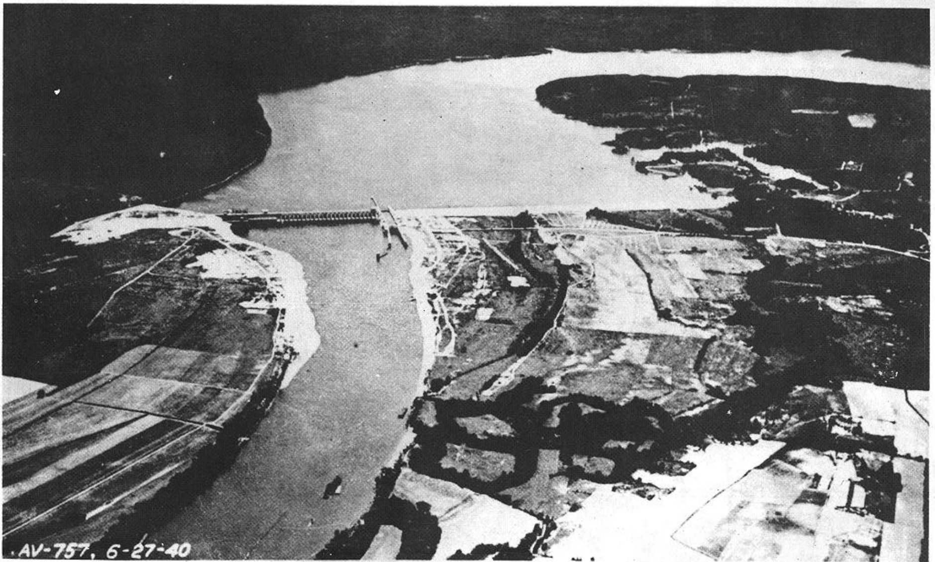
Figure 11. Aerial photo of Pickwick Landing Dam.
